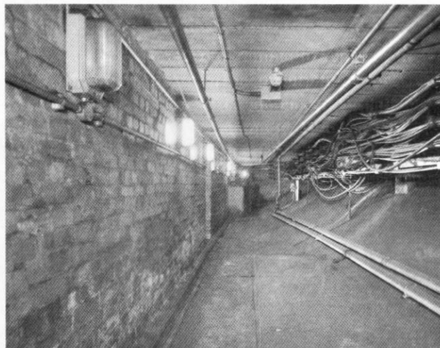
All that now remains of the deep-level District Line tunnel. Photo by Nick Catford
